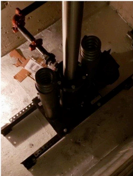
Completed Jack Unit
